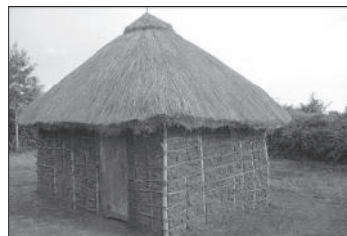
Fig. 4: Completed house before finishing touches are made on the walls, which are continuously smeared with red mud and cow dung for protection from pests and aesthetic purposes. Originally the doors were made from woven reeds and tough animal hides, but currently iron sheets are used for security purposes (Ojoo, 2009).
