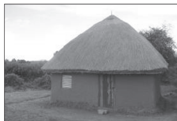
Fig. 5: After touches – cow dung and red mud decorations on the walls. Roof thatching is an art and a good roof would be flawless and able to withstand rainy and windy conditions for over six years (Ojoo, 2009).
